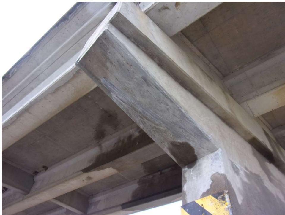
Photo 4: Underside of Pier Cap Cantilever
