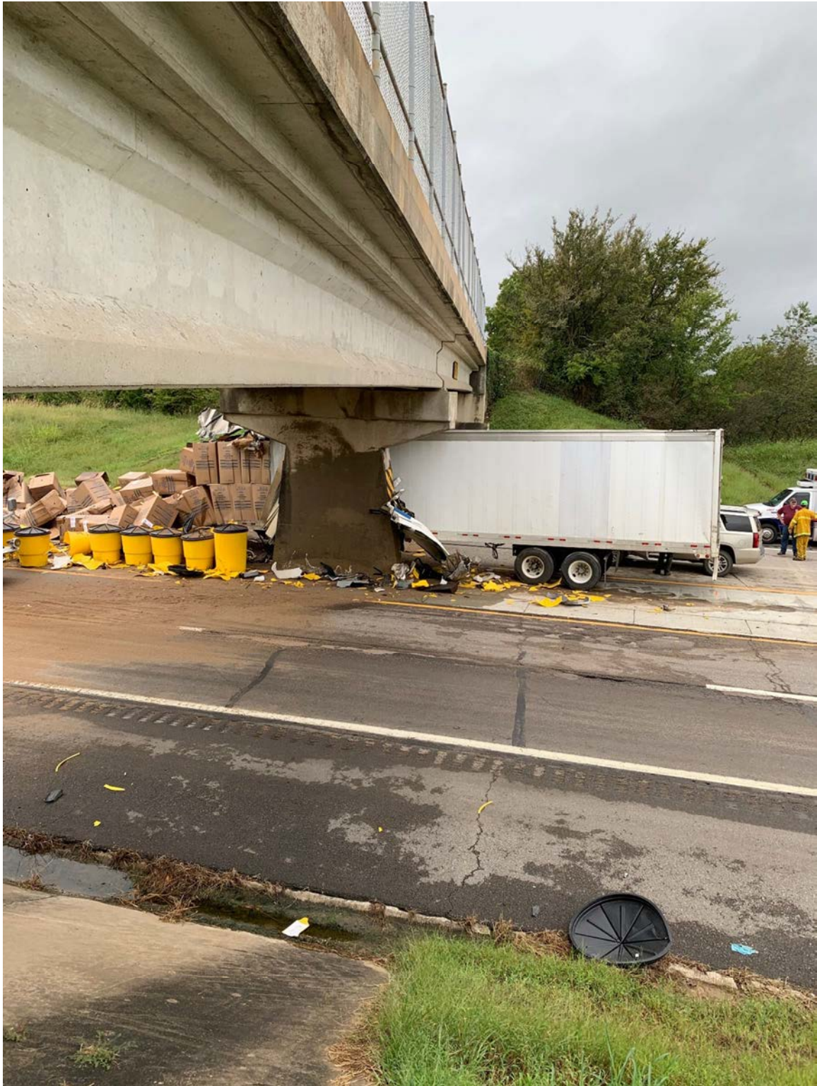
Photo 2: Center Pier (Facing West)
