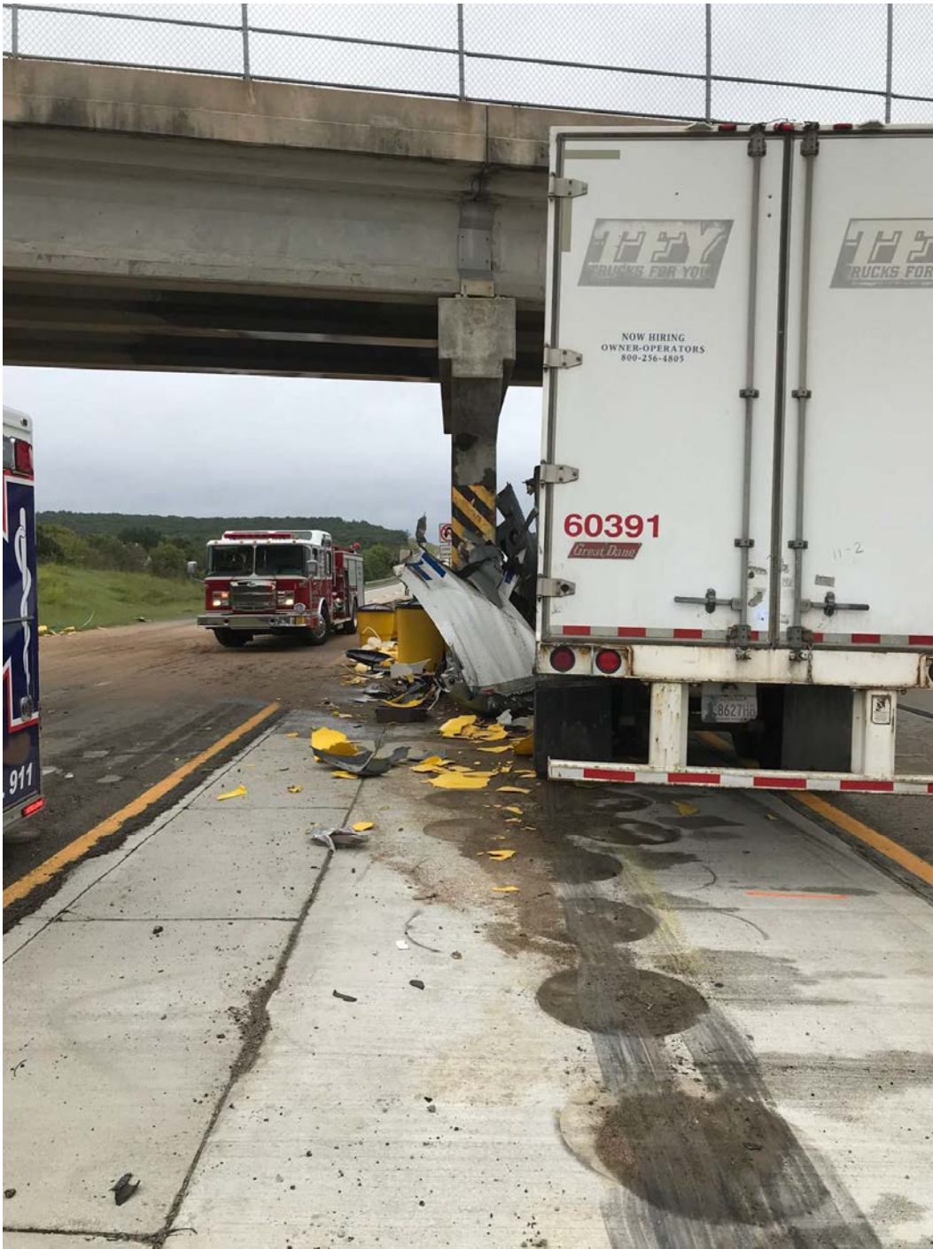
Photo 1: Bridge 50.33 (Facing South)
